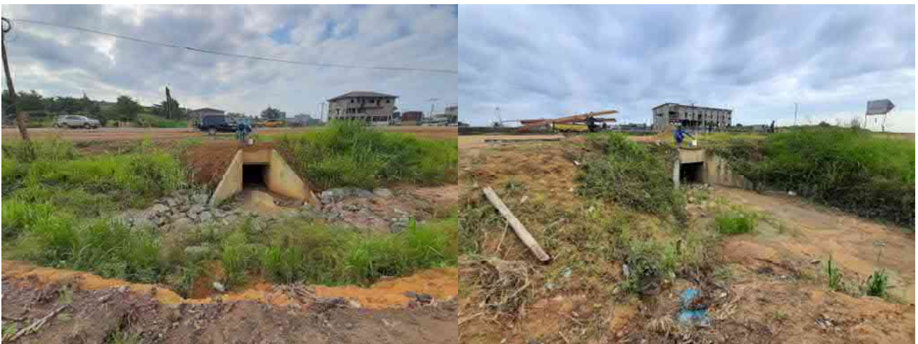
FIGURE 2-24: EXAMPLES OF INSTALLED HYDRAULIC STRUCTURES
