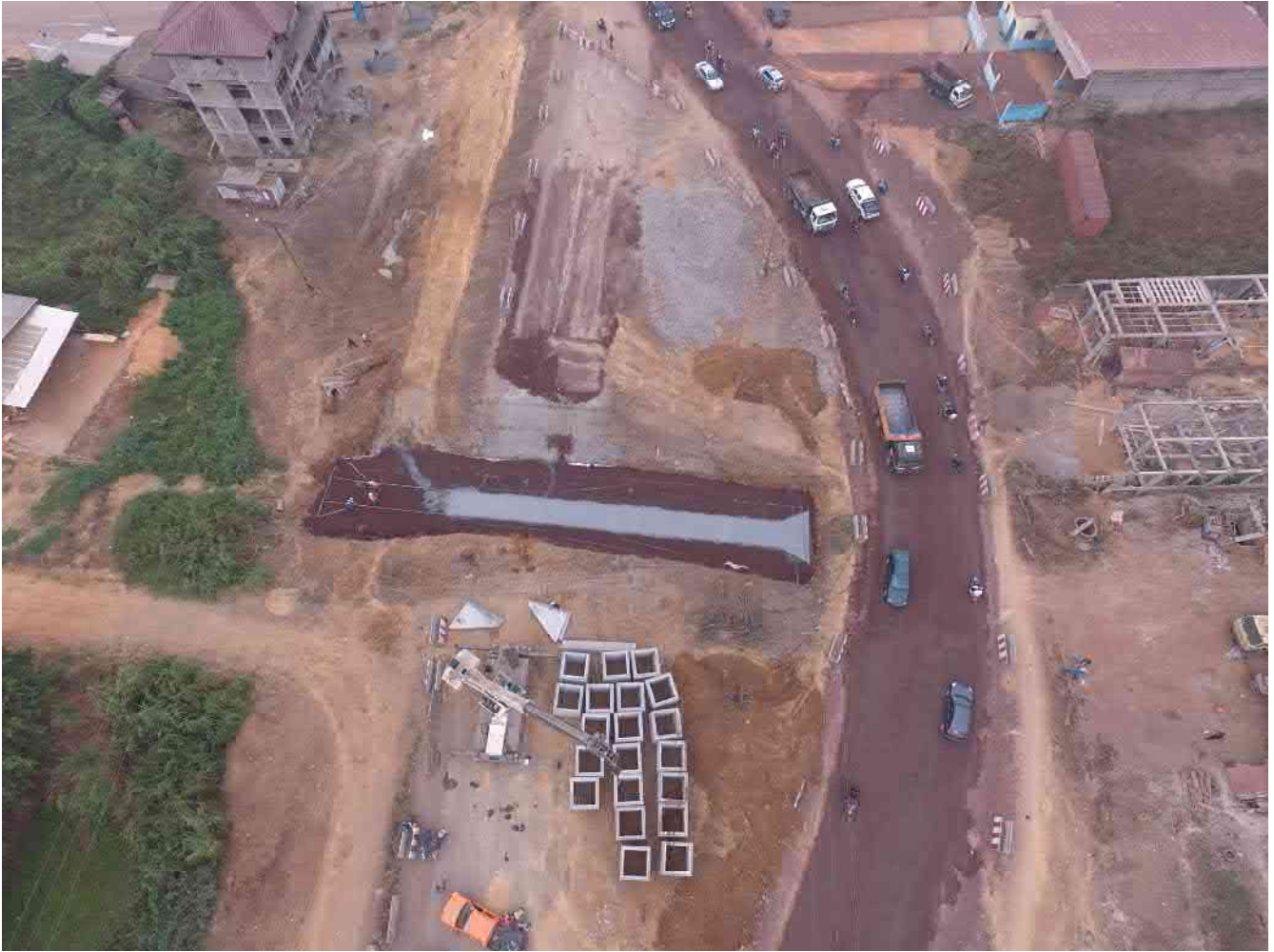
FIGURE 2-23: INSTALLATION OF HYDRAULIC STRUCTURE AT PK 13+282
